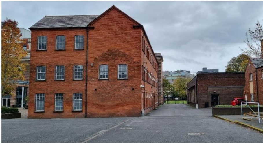
Figure 1: Listed W-Block proposed to be demolished
